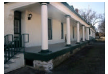
Administration Bldg Exterior 2010
